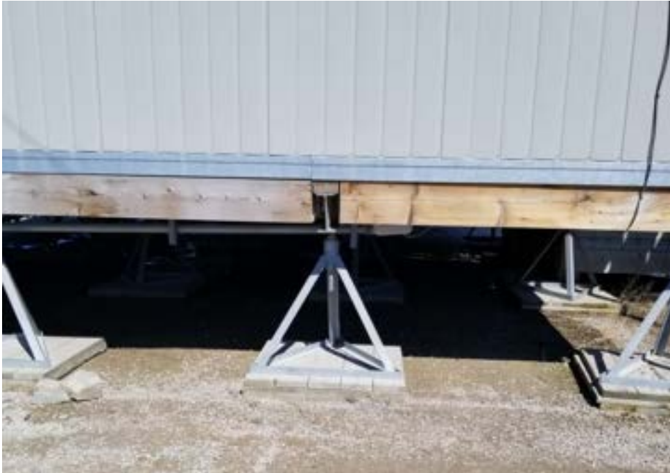
Figure 10 Adjustable screw jacks. Source: Qillaq Construction
