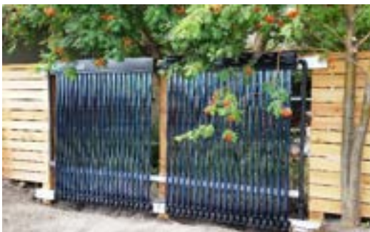
Figure 12 Solar thermal collectors as part of a fence. Source: Simple Solar Heating Ltd.
