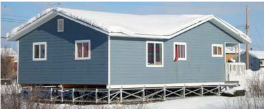
Figure 7 Triodetic foundation. Source: Multipoint-Foundations
